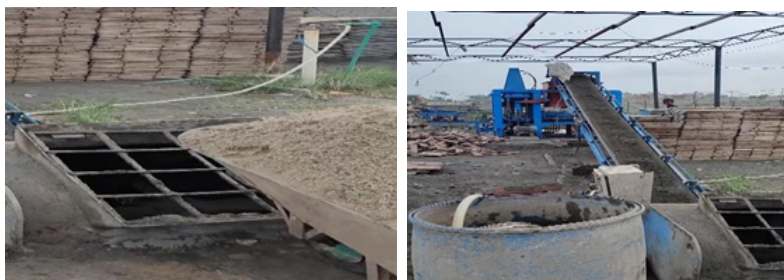
Figure. 2(a) Mixing the material in the mixture (b) Conveyor belt carrying the mixture
